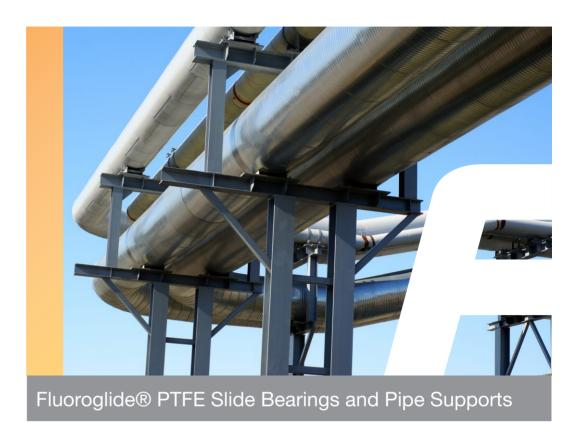
Fluoroglide® slide bearings are superior to conventional expansion plates, rollers and rocker arms, accommodating expansion, contraction and other reciprocating motions of any structure that moves as a result of thermal, seismic or differential forces.
